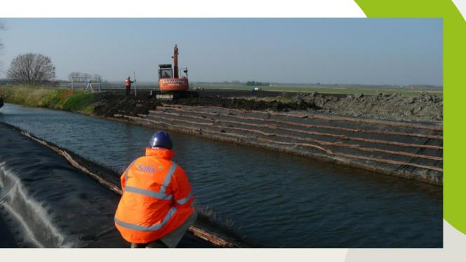
The liner prevented stakes being used and created a slippery surface for soil placement. Therefore, a woven loop geotextile was used over the liner in order for Coir Rolls and brushwood fascines to be tied onto the loops.
