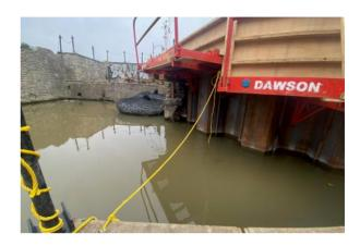
We backfilled the sheet piles with a self-compacting gravel up to the underside of the formation level for the capping beam, leaving a gap for shuttering installation. Blinding concrete was installed landside to provide us with our level for the concrete capping beam shuttering. To ensure that the gap between the new and existing structures was fully sealed, we used mass pour concrete.
