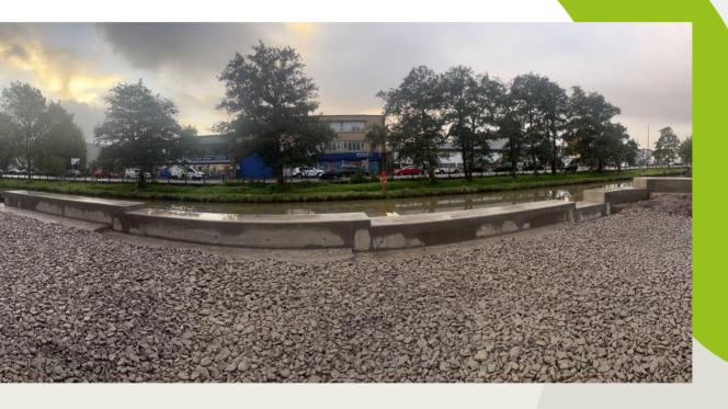
During the development stage we designed a cantilever, sheet piled wall enabling removal of any potential footing or drainage clashes associated with the original anchor block design brief. Achieving a design life of 60 years.
