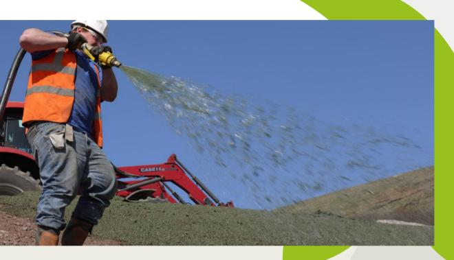
HydraCX is a hydraulically applied erosion control product that protects slopes against soil and seed loss from heavy rain and wind from day one of application. It is 100 per cent natural, consisting of reclaimed cotton and straw fibres, and is an effective alternative to a biodegradable rolled erosion control coir/jute matting or netting solution.
