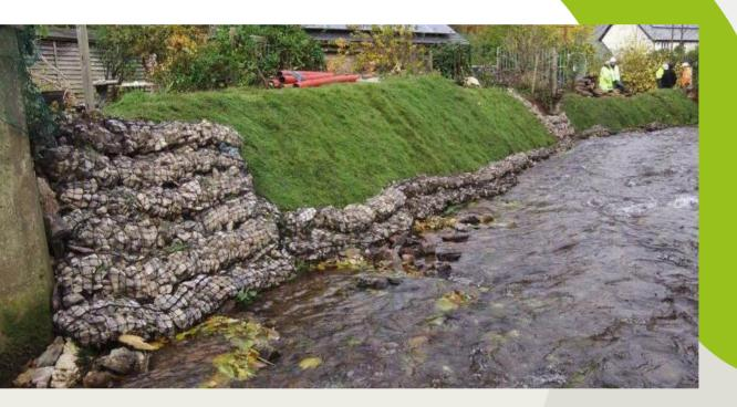
A forty metre section of the river which had timber piled revetment running between properties required urgent attention. These piles were at the end of their working life and new erosion protection was required. The site was constrained on both sides and as such a conventional system was not feasible.
