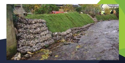
They were placed to provide "engineering" resistance to flow and also to create natural features with habitat value. They are sewn together where they touch to create one mass, either in line or where stacked up the slope.
