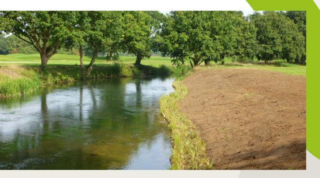
Working with Global Golf Builders we regraded the riverbanks, added in Coir Rolls and Coir Pallets and hydroseeded the soil.
