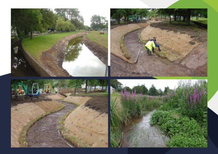
The stream banks were seeded with a local wildflower mix and protected with fully biodegradable erosion control blankets (C125BN). The new channel is an effective flood reduction measure, whilst providing a valuable ecological habitat and a landscape focus in the town.
