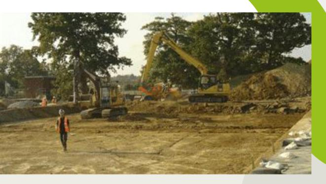
A 2000m2 reedbed involved a composite approach using both a Sub Surface Flow (SSF) gravel reedbed and a large floating/rafted reedbed in order to meet the treatment criteria and retention times within a limited land footprint. As SSF reedbeds can blind over a relatively short period of time the reedbed was designed as an overland flow wetland so that performance would be guaranteed longer term.
