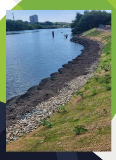
Working from the top of the bank, using a JS220 15 m long reach excavator, we cleared vegetation from the full length of the bank, with off-site removal, in preparation for the installation work. We then set the line from the toe to the existing boundary.
