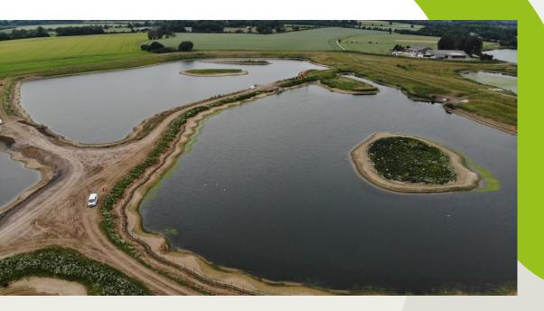
Wetlands were excavated as part of a large, new retail development near Doncaster. Once excavated, the embankments suffered from significant erosion due to sandy soils and wave action. The structural integrity of the embankment was at risk, which would lead to failure of a bund and continued erosion.
