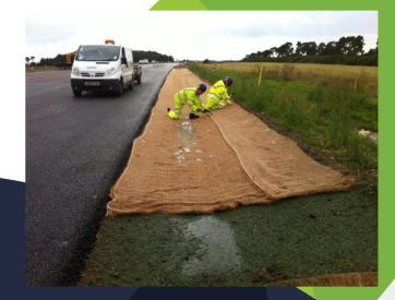
A tough grass selection was added to the straw, cotton, polymer and tackifier mix, these plants could withstand the level of pollution being washed off the road.
