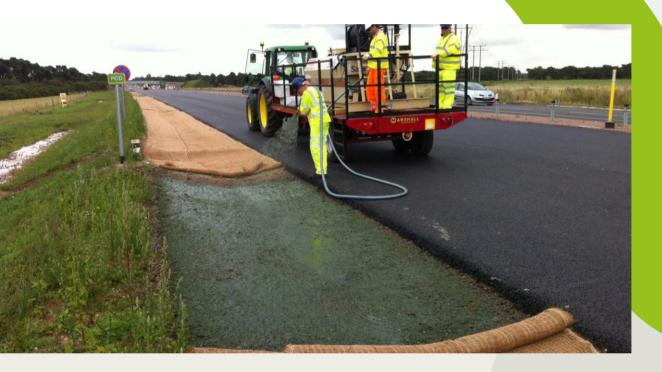
The new soft engineered 'Green Swale Grass Channel' attenuates road runoff water, filters suspended solids, and traps hydrocarbons and heavy metals, significantly improving water quality.
