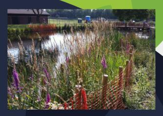
The soft bank protection was broken with areas of timber capped sheet pilling to offer lake side access to this important amenity lake.
