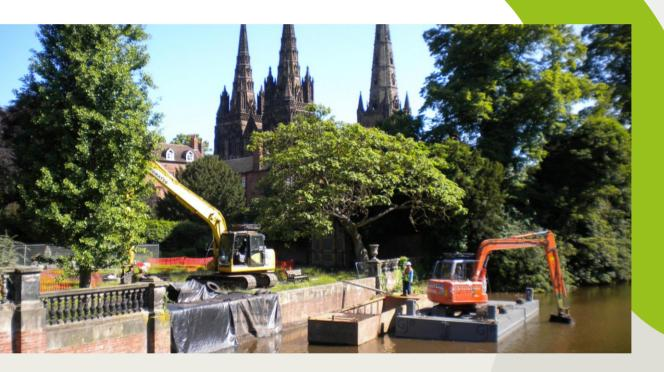
The lake was heavily silted with sediment deposited from the brook and with many years of decaying leaf litter. The lake was created many years ago by filling in over peat bog which left the lake with soft and rapidly eroding banks of made ground.
