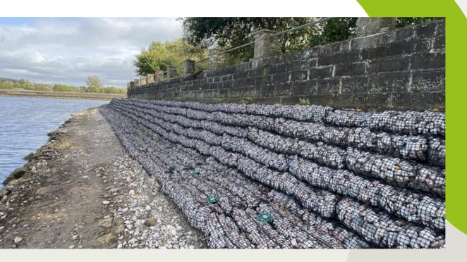
The project involved the installation of a durable rock mattress revetment to replace a failing retaining wall and create a stable, long-term platform for angling, including wheelchair-accessible areas on both the north and south shores.
