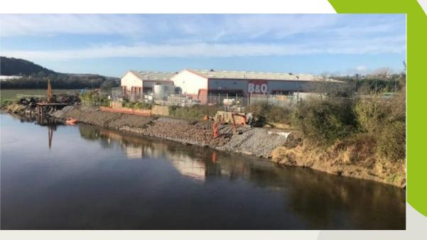
Cbec eco engineering conducted a range of surveys to allow detailed hydraulic modelling to inform the best design solutions. The final design was based upon the known shear stress at a 1 in 200-year flood event.
