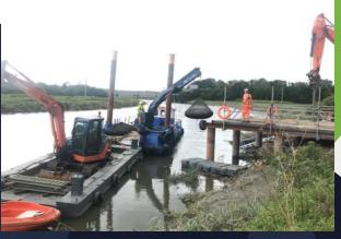
AquaRockBags were installed at the eroded toe of the falling riverbank. Brushwood was then applied to the surface of the newly formed slope.
