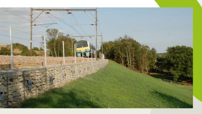
The geotechnical issues of ground stability were resolved using soil nailing. The surface erosion was solved by using VMax C350. C350 is a composite Turf Reinforcement Mat (TRM) and was installed over prepared seeded topsoil.
