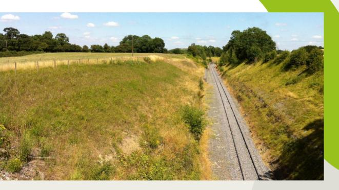
Due to the high stone content on the surface, Salix requested the main contractor to rake the top surface area to expose the fines below. We then sprayed this with HydraCX, our hydraulically applied erosion control blanket. Some areas were nailed and rock netted.
