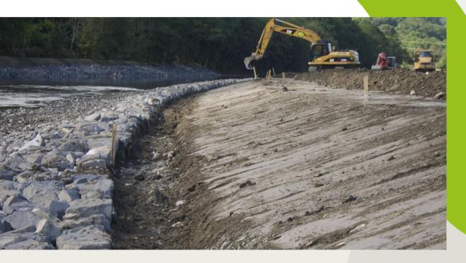
Difficult site access created problems for using large blockstone. Salix replaced part of the blockstone armouring with VMax P550.
