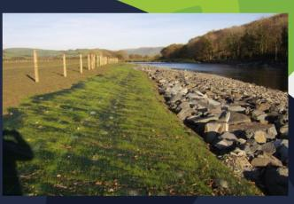
The works were carried out at the end of October, which meant that the P550 remained only partially vegetated throughout the winter months of frequent flooding. By the end of the following Spring, there was no soil erosion and a good rate of vegetation establishment.
